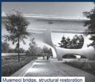
Musmeci bridge, structural restoration
