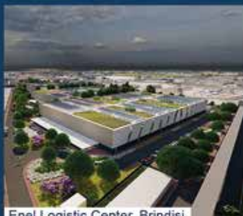
Enel Logistic Center, Brindisi
