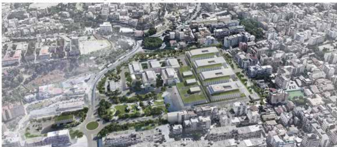
New "Morelli" Hospital - Reggio Calabria
